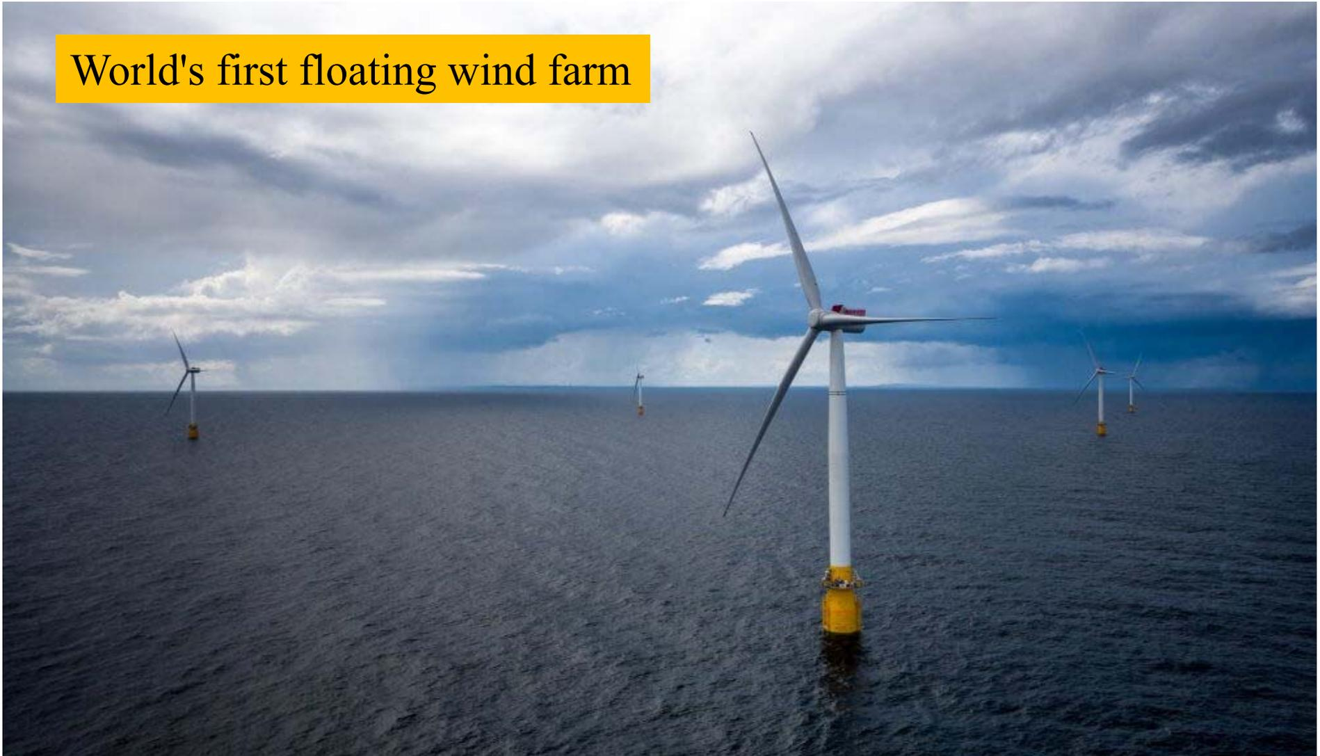
Three months after deployment, the world's first floating wind farm surpassed performance expectations, according to its operator, Statoil. The five-turbine, 30-MW Hywind Scotland Pilot Park — situated 15 miles off the Aberdeenshire Coast — operated at 65% of its maximum theoretical capacity last November, December, and January, the Norwegian energy company said.
